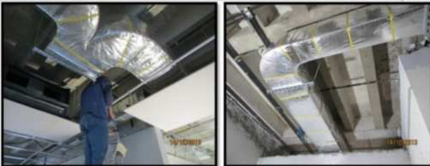
HVAC works : Install A/C Duct
