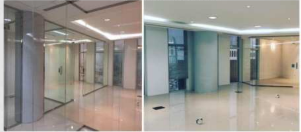
Glass, Electrical and tiles works
