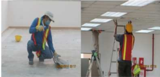
Removing carpets and Ceiling
