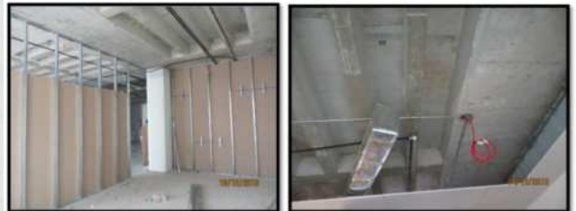
Electrical works : Install Conduit pipe and wire for power & Lighting
