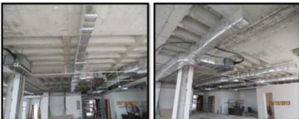
HVAC works : Install A/C Duct
