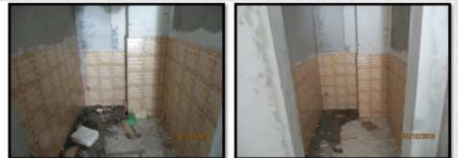
Civil works: Installation ceramic at W.C
